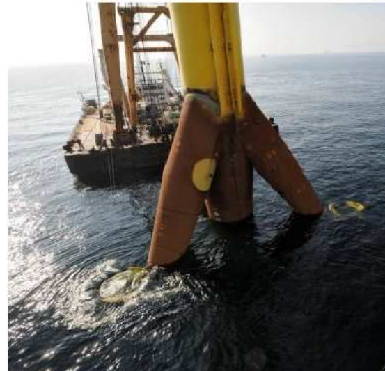
Tripod foundation lowered to seabed
