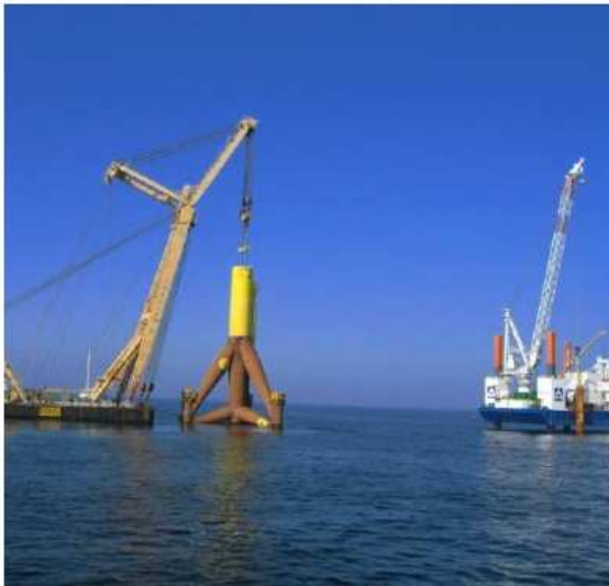
Heavy-lift crane ship on site
