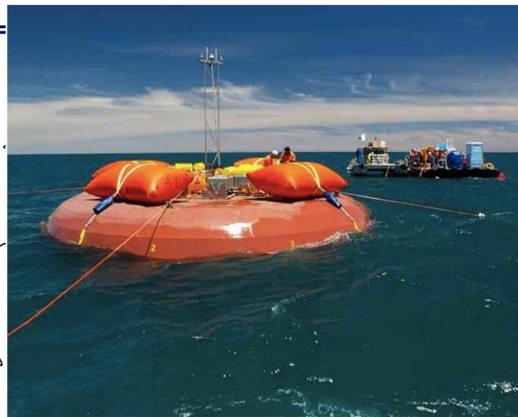
CETO 5 unit during installation at the Perth Project site
